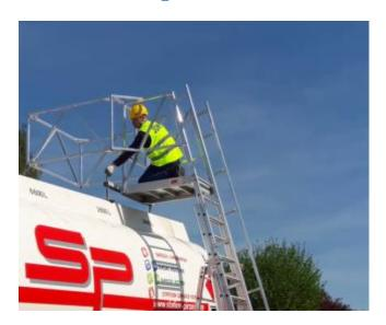
After this action, the structure is ready to be used within the perimeter of its upper cage:
