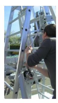
3) Lower the mobile ladder with the winch. Maintain the brake open with the handle just to let one rung pass it and then let go of the handle so that the brake balances back to its blocking position. This is done as a safety measure against an unexpected ladder drop-down, e.g. in case of a sudden cable rupture.
